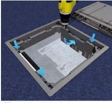
**7** | The mounting of lock-in leads The separately delivered lock-in leads can be inserted into the installation unit from the top and tightly screwed. For a flat installation the 50 mm lock-in lead must be used.
